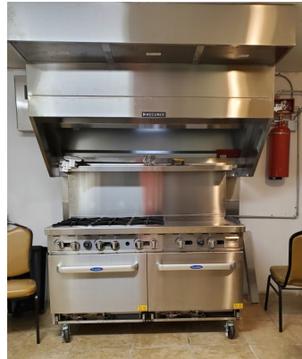
Dining hall with new commercial stove, hood vent, and fire protection
