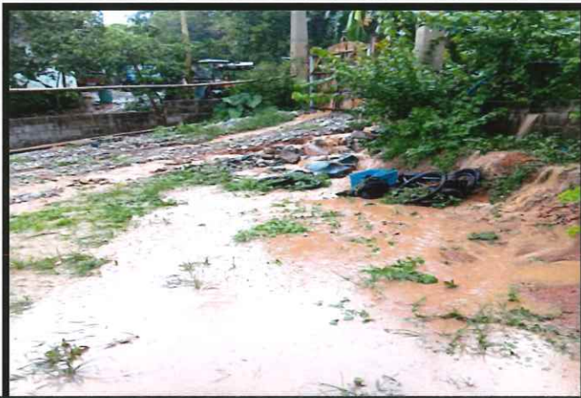
The proposed parking lot was damaged due to heavy rain, but no discouragement, God will help us. The work may resume next dry season.
