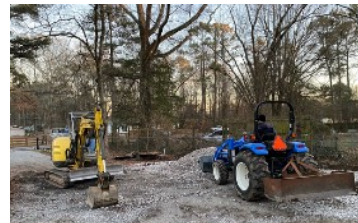
Site prepared in September '22
